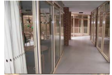
Glazed internal corridor walls
