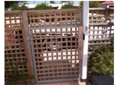
External gate fitted with keypad & electronic strike with auto release.
