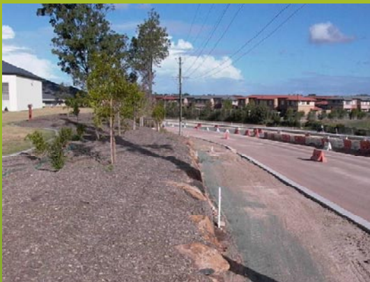
Resident external courtyard area with no fencing to prevent access to 1.5m fall to main road
