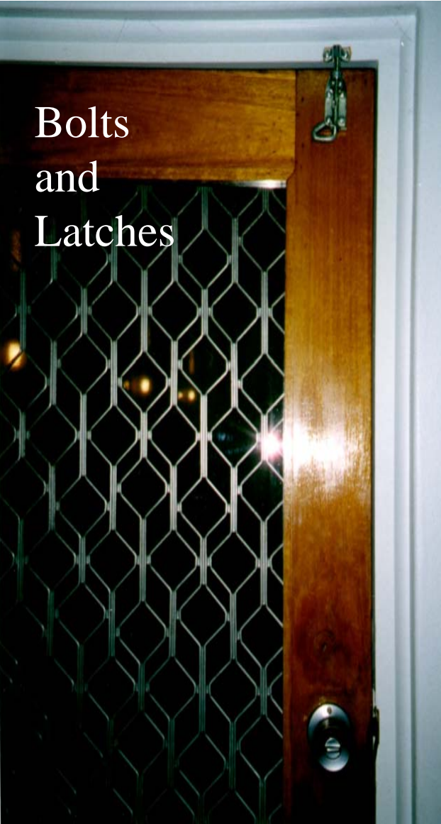
Exit door swings inwards and security screen
