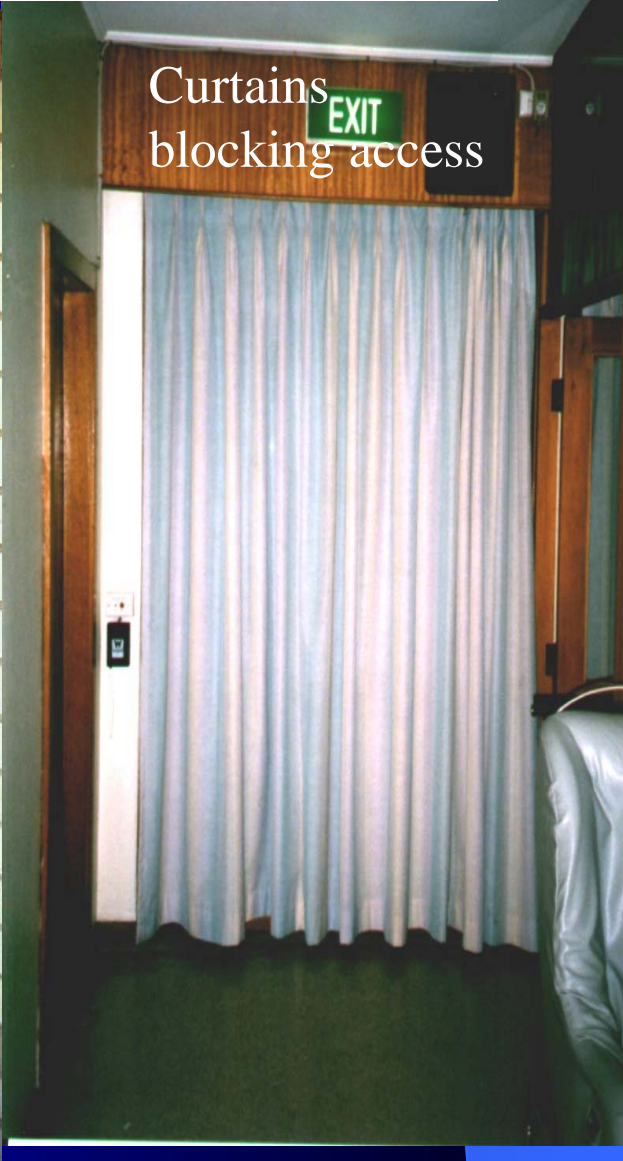
Exit door swings inwards and security screen
